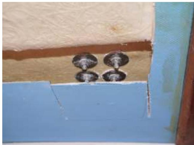
*Bolts securing the 'stand-up' block on the port side, which leads No2 reefing line to the deck organiser*
